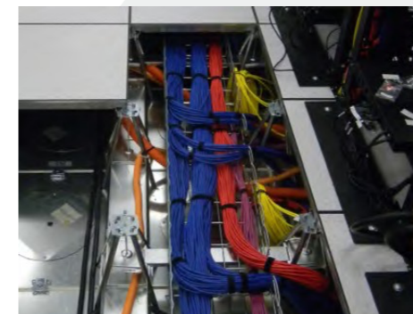
All cabling is easily installed in cable trays without disturbing airflow.
