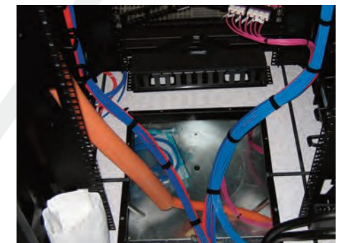
Easy to access cut outs without losing airflow or requiring gaskets
